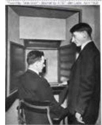
Frank Gray and A. L. Johnson in laboratory bench. Behind the glass panels on sides and top are the photo-electric cells.
