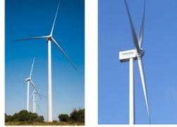
Large three-bladed horizontal-axis wind turbines (HAWTs), with the blades upwind of the tower produce the overwhelming majority of wind power.
