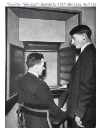
FRANK GRAY and A. L. Johnson in television booth. Behind the glass panels at sides and top are the photo-electric cells.
